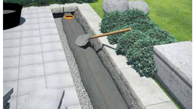
Fill with concrete and compress to foundation.
